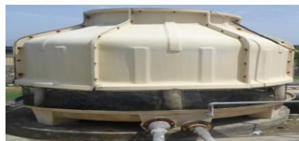
Fig. 14. Cooling Tower
